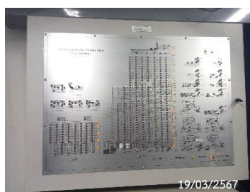
Graphic Annunciator Fire Alarm System
